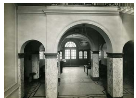
The original front doors (interior),
